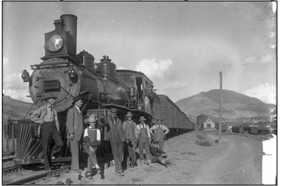
Steam locomotive and train at Paonia in about 1911.
